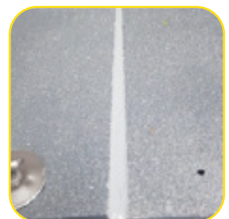
4. Once the sealant has dried, the floor is ready for use
