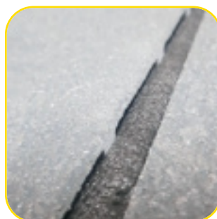
2. Insert the expansion joint cord
