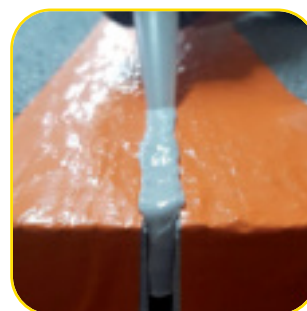
3. Secure the edges of the gratings with tape and fill the gap with polyurethane
